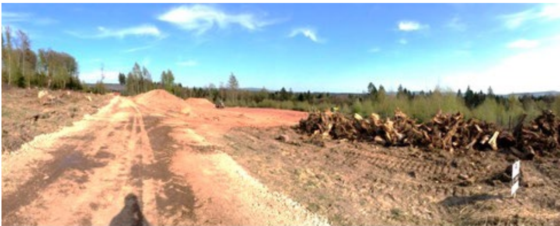
Fig. 24: windpower constr. site in the Kaufunger forrest nature park (Hessen 2016)
