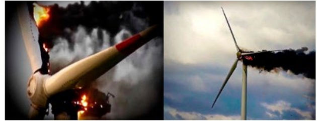
Fig. 38: Burning wind power plants
