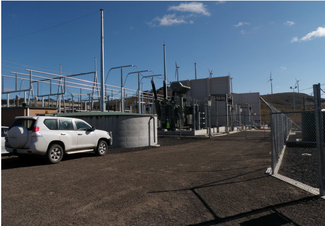
Substation with concrete barrier shielding
