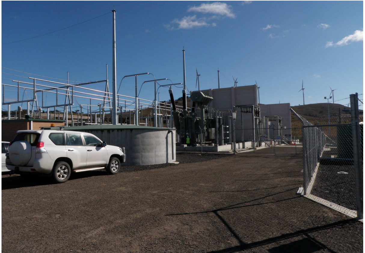
Substation with concrete barrier shielding
