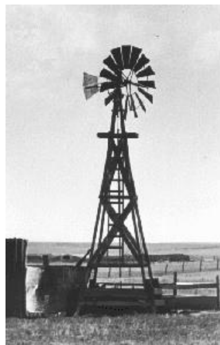
Figure 10: Steel-bladed water pumping windmill - America Mid-West late 1880s.
